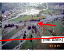
Aerial view of debris-flows Modane (left bank)
